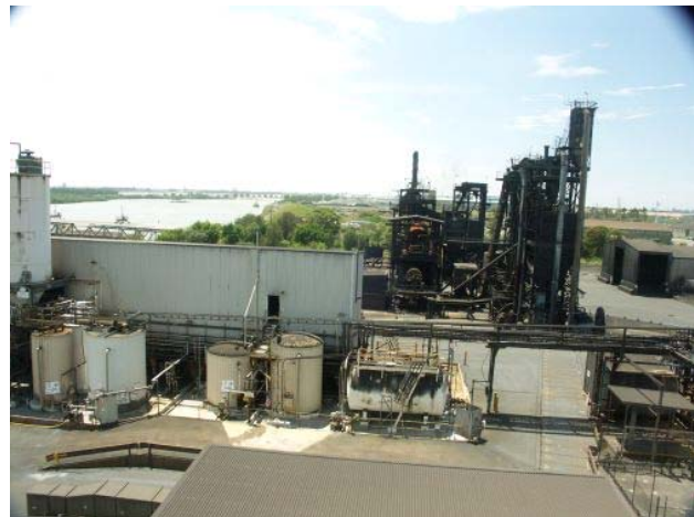
Figure 1: The Refractory Unit and reagent storage, viewed from the west.
