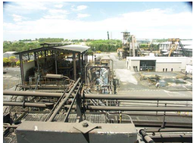
Figure 4: The filter shed of the Hydrometallurgical Unit
