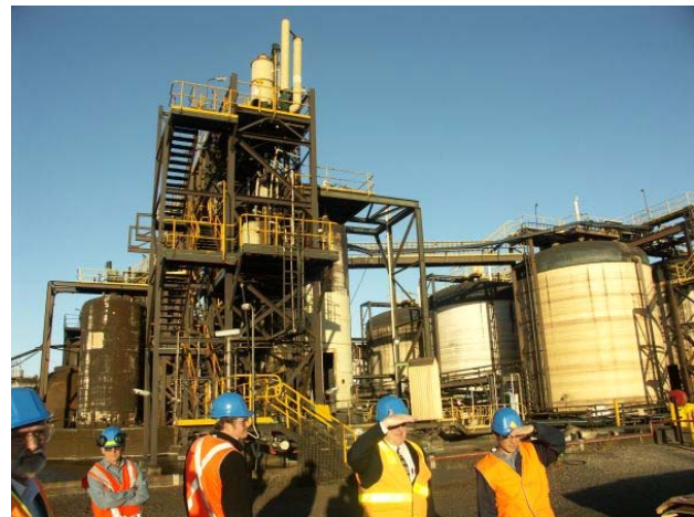
Figure 2: The leach and purification sections of the Hydrometallurgical Unit
