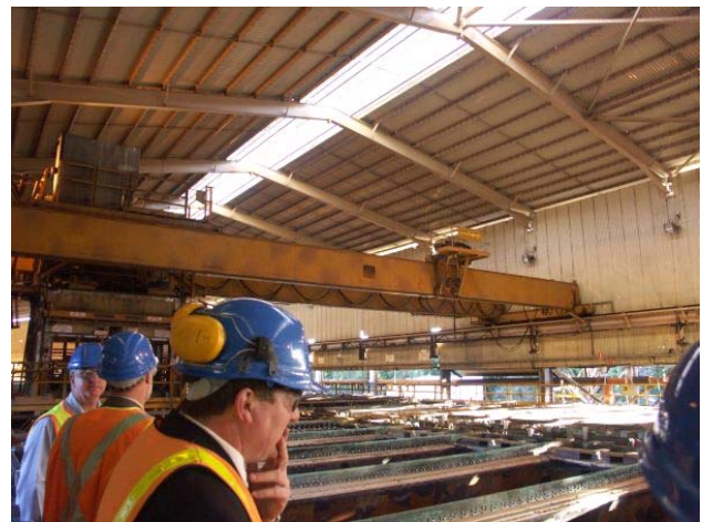
Figure 5: Inside the massive electrowinning tankhouse of the Hydrometallurgical Unit
