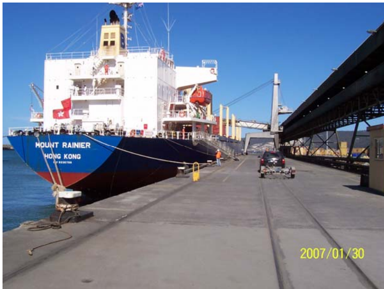
Above – The “M.V. Mount Rainier” dockside at the Port of Burnie showing the concentrate conveyor and bulk loader at right
