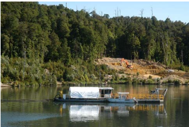
Above – The dredge in operation on the Hellyer tailings dam.
