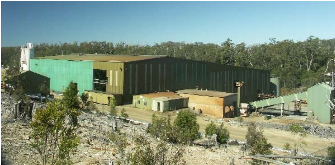
The Intec Hellyer Mill, viewed from the 'run of mine' ore pad to the south-west of the plant
