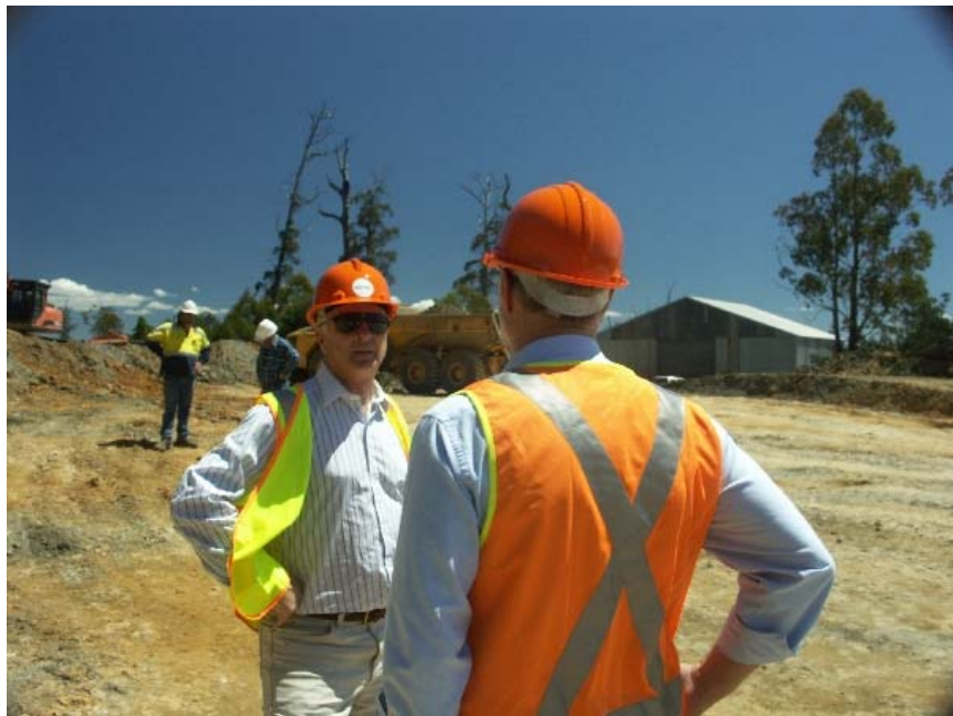
Philip Wood (Managing Director & CEO) with John Moyes (Technical Director) at the bunker storage pad. The receiving shed is shown in the background.
