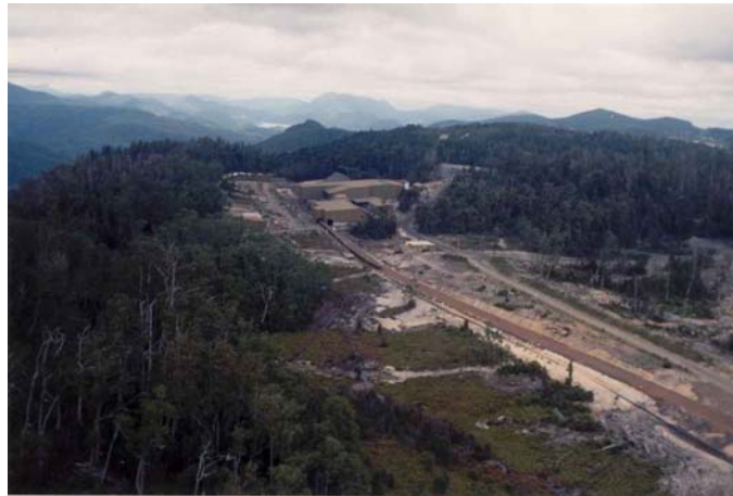
Figure 3: Hellyer Mill and infrastructure.
