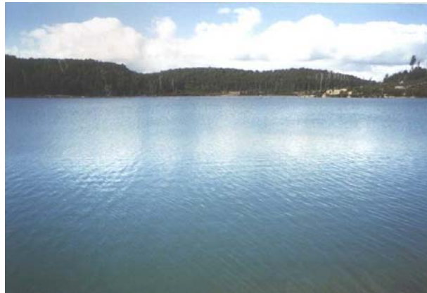
Figure 2 Hellyer tailings dam
