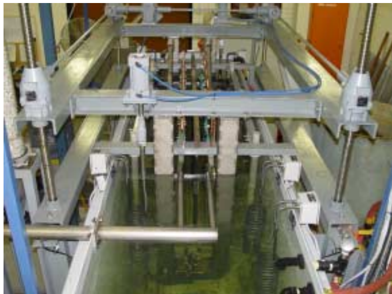
Figure 1: EW cell under construction at the University of Sydney as of January 2003.
